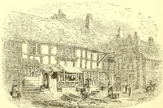
[House in Henley Street, about 1820.]
